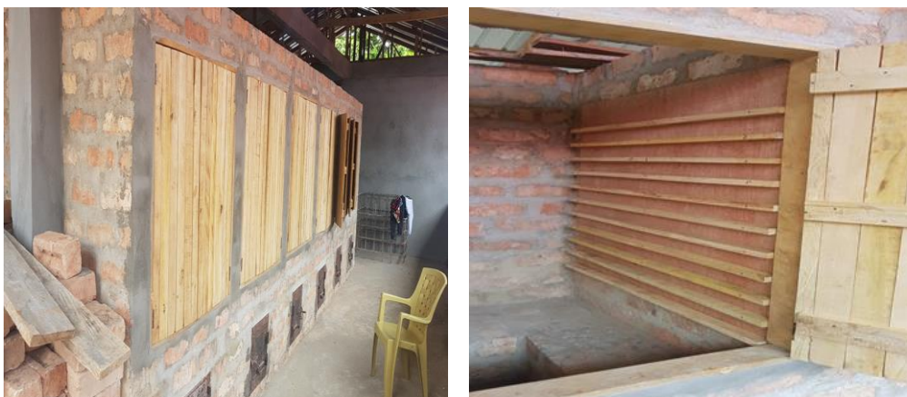
Figure 3. Cabin smoking kilns constructed in Sierra Leone (Gbla, 2020).
