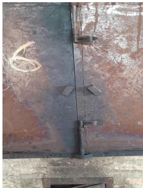
Figure 28: Metal door with locks
