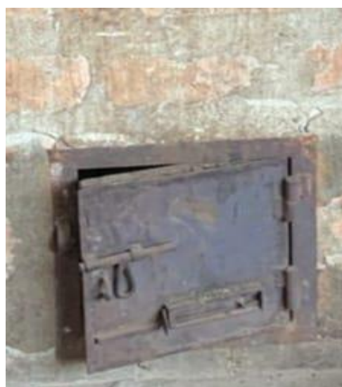
Figure 11: Closed oven during smoking (a); Fire chamber door with the air valve and lock (b).
