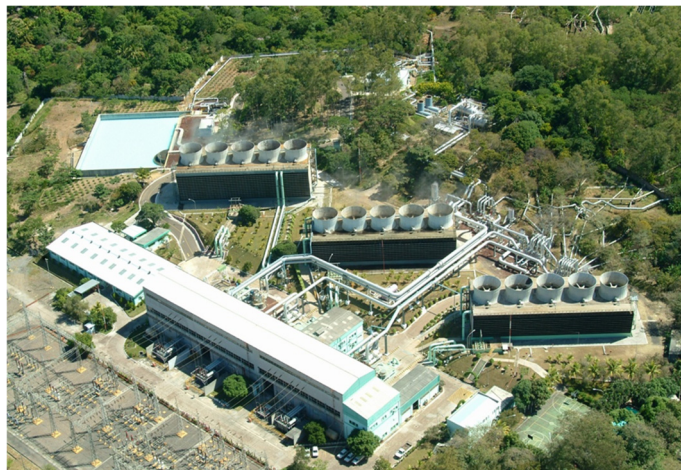
FIGURE 3: Ahuachapán geothermal power plant (LAGEO 2020d)
